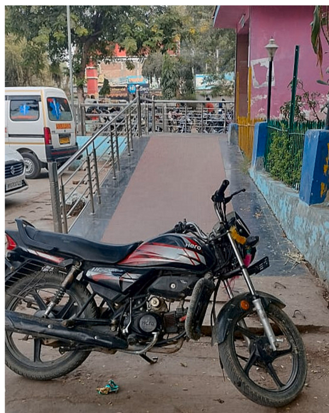
Image 5. Obstructed ramp. An external ramp of the hospital with proper railings on one side, but not the other. The ramp is obstructed by a 2-wheeler parked in front of it.
